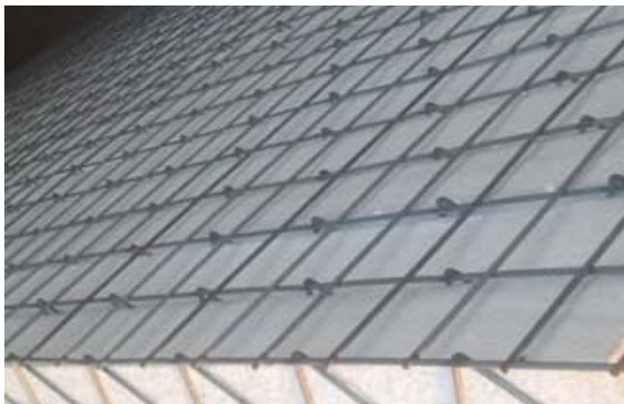
3D panel - bend welding
